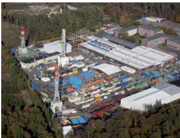
Bentec's production site in Bad Bentheim, with four rigs under construction
